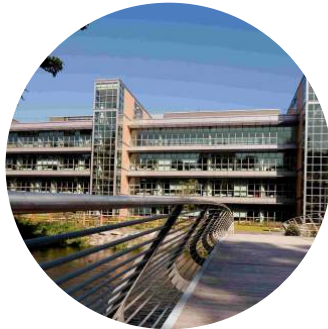
Western Gateway Building (WGB)
